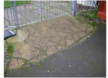
Entrance – Slanted Paving
